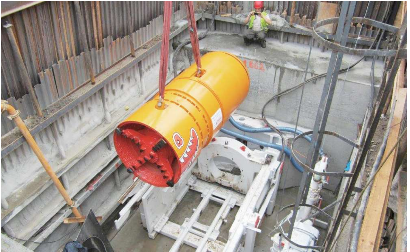
Unclemole lowering down to shaft
